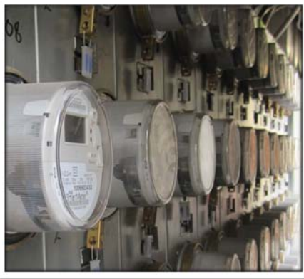
Challenging Metering Configurations at a Multi-unit Dwelling
